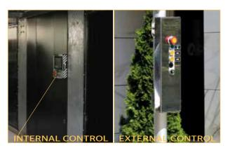
2 DOUBLE SPEED According to the 2006/42 / EC directive; the driver can use the control panel from inside the cabinet if the speed is less than 0,15m/sec. Optionally, it can be controlled from outside the cab for higher speed.
